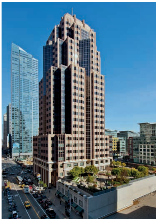
100 First Street og 303 Second Street, San Francisco ↑
